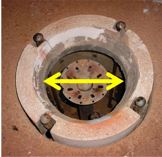
Figure 3 Burner tile throat which creates an orifice to meter the combustion air flow.
