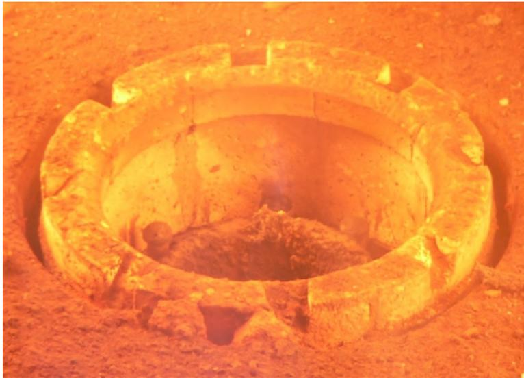
Figure 16 Burner tile installed upside down.
